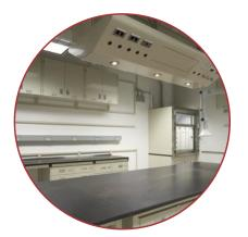
Flexible Solutions - Ideal for use with mobile carts and tables because instruments and equipment can be easily connected to the service supply as needed and simply moved out of the way when finished.
